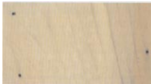
Typical dark rimmed bore holes of Ambrosia beetle damage in sapwood
