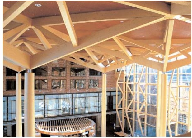
Figure 4 Lahti Sibelius Hall, Finland. An example of internal structural glulam. Composite glulam and LVL both in spruce.
