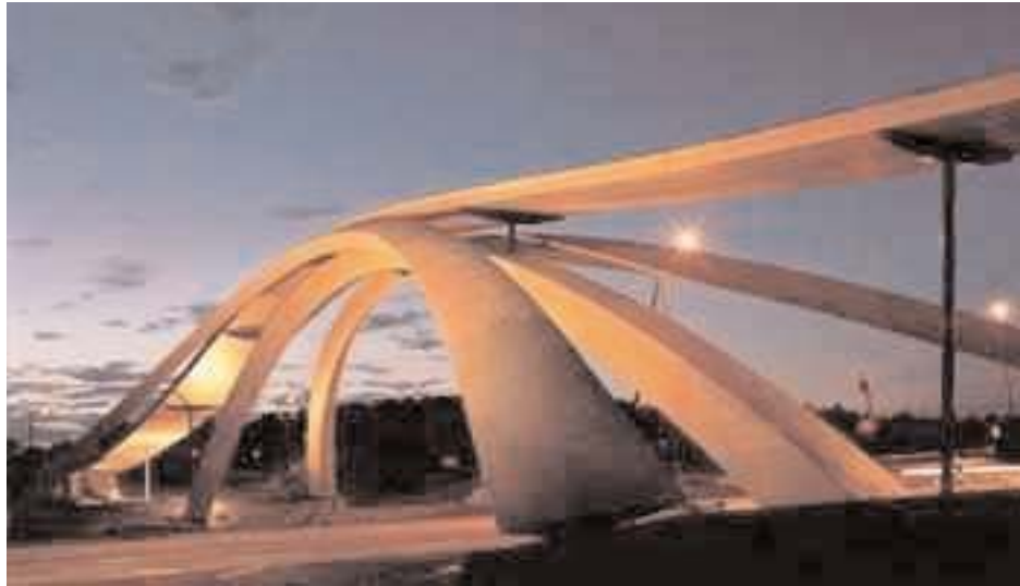
Figure 1 This striking glulam bridge, near Oslo in Norway, is based on a Leonardo da Vinci design dating from 1502. Vision: Leonardo da Vinci, Vebjørn Sand Architects: Selberg Arkitektkontor Engineers: Reinertsen Engineering Glulam fabricators: Moelven Limtre. Photograph: courtesy Terje Johansen Further information: www.vebjorn-sand.com/thebridge.htm
