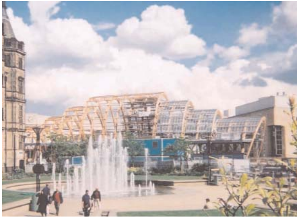
Figure 3 Winter gardens, Sheffield. This larch glulam structure forms part of the city's current regeneration process. Architects: Pringle Richards Sharratt Structural Engineers: Buro Happold
