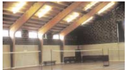
Figure 2 Ply-box portal frames
