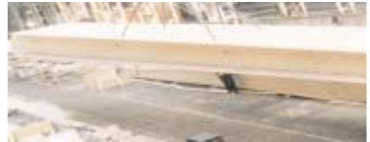
Figure 1 Stressed skin panels, 24 m long; clear span 21 m Photo: Cowley Structural Timberwork Ltd
