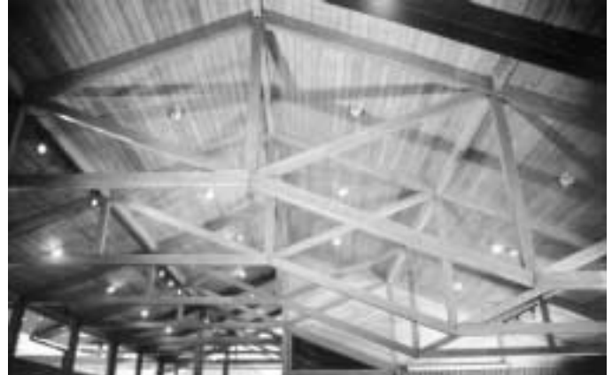
Oak trusses. Photo courtesy Cowley Structural Timberwork Ltd
